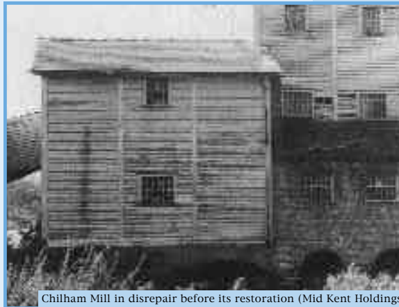
Chilham Mill in disrepair before its restoration (Mid Kent Holdings)
